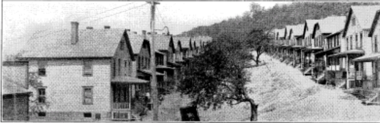
LOW COST FRAME HOUSES. MIDLAND Tenants of these double houses are foreign laborers and mechanics. They pay $12 per month for five large rooms, inside toilet, running water, gas, electric light, and fireplaces. The street is shown still in process of construction
