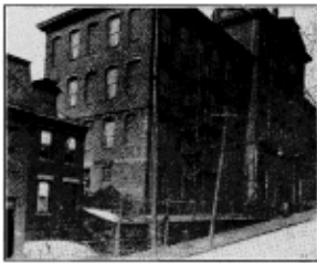
Exterior: Showing drain pipes emptying on sidewalk
