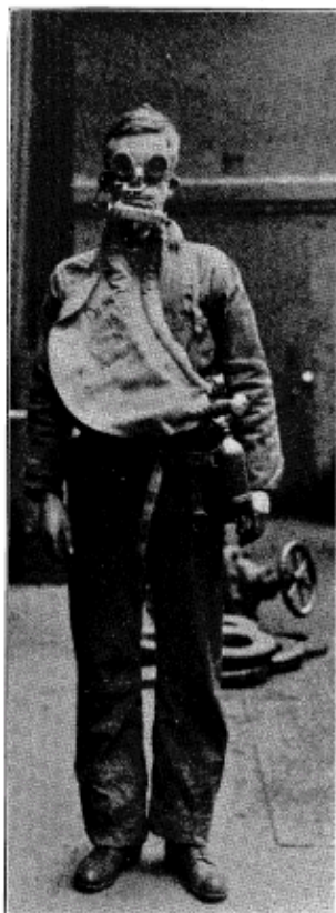
OXYGEN HELMET Repair man equipped against gas poisoning ready to enter a blast furnace. The equipment used is that developed in mining, applied to furnace work by the Carnegie Steel Company since 1911
