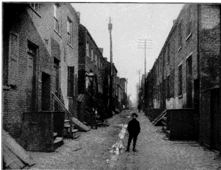
ALLEY DWELLINGS The cellars used for living purposes: Mulberry Alley from the corner of 13th Street
