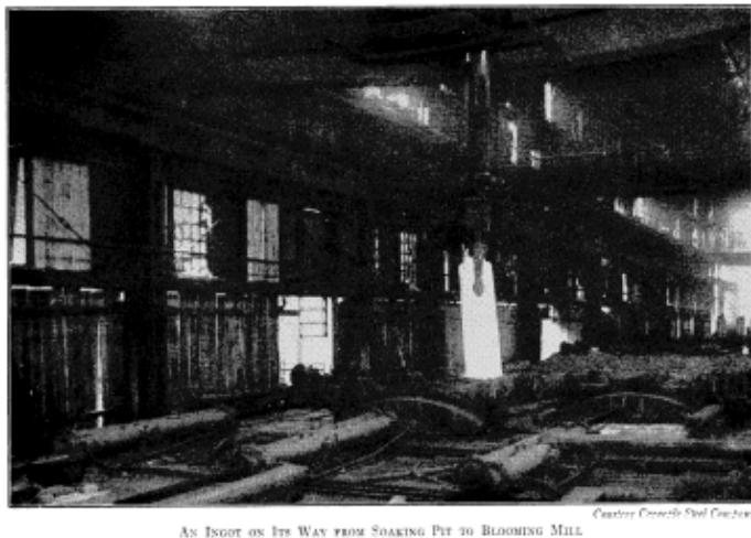
Figure 25 : An Ingot on Its Way from Soaking Pit to Blooming Mill et Plate Mill (The Steel Workers, pp. 44 et 56).
