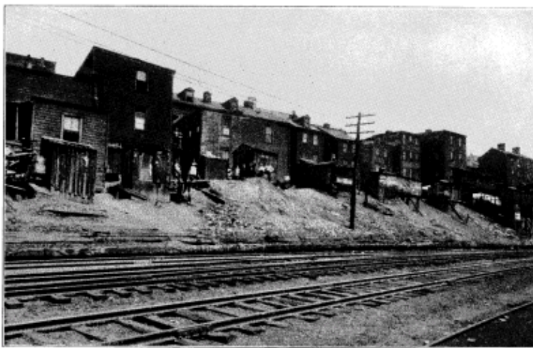
A HILLSIDE BATTERY OF DISEASE Thirteen dry uncovered vaults are shown in the length of the picture. Waste water drains down over the embankment, alongside the tracks where the through Baltimore and Ohio passenger trains set the dust awirl. The vault next the end at the left is all that is supplied to three houses, sheltering eight families
