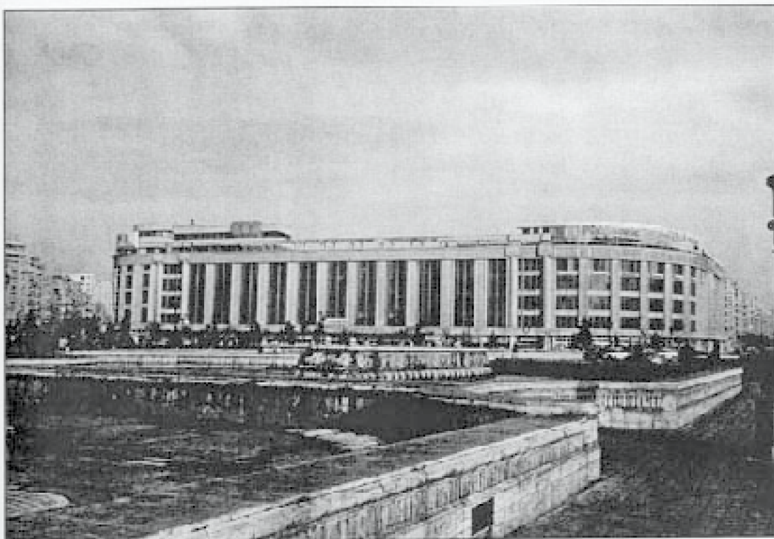
Facade centre commercial Unirea.
